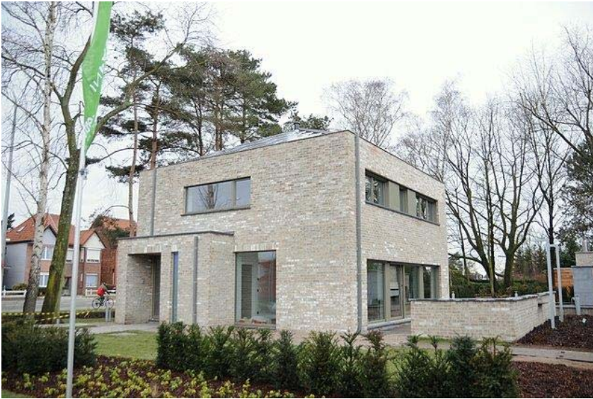
Massive passive house in Lochristi, architect: C. Debrabander, photo: PHP
